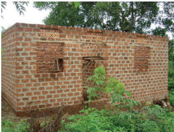
House needing completion
